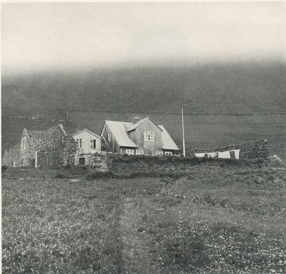
BRACED STONE WALLS DEFLECT THE VIOLENT WINDS
